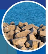
STEEL slag and moulds are used in the manufacture of coastal marine blocks, tetrapods, biorocks and gabions to improve the ocean environment and protect the shoreline from erosion.
